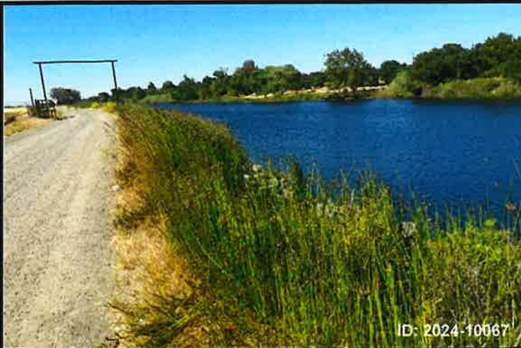
Photo 1: Vegetation Growth - Dense vegetation including grasses and weeds up to 3 feet tall along waterside slope. Inhibits inspection.
