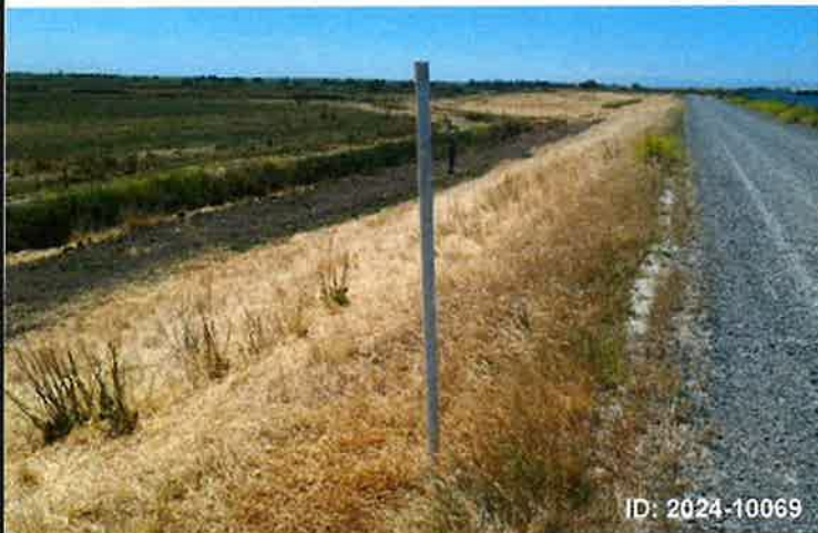
Photo 3: Encroachment - 2-inch diameter PVC pipe for piezometer well at landside hinge. PVC pipe extends 5-feet above ground.
