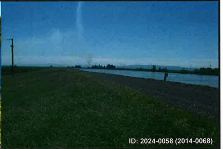
Photo 2: Settlement - Approximately 0.5- to 1-foot dip in levee crown elevation. Extends approximately 200-feet.
