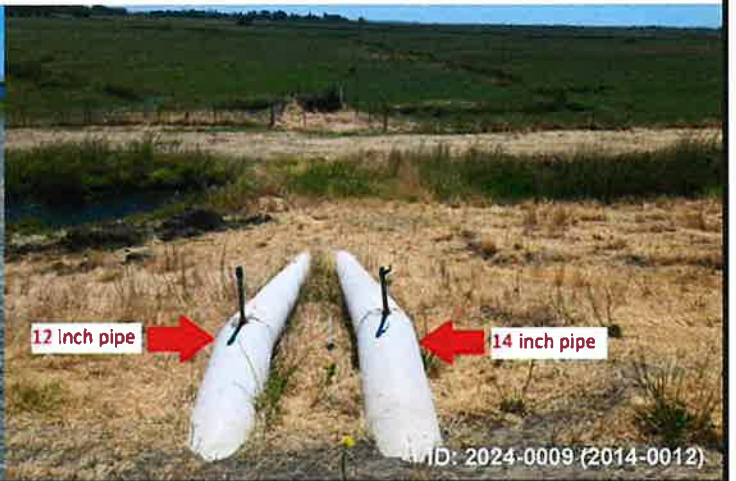
Photo 4: Encroachment – Landside view of two metal siphon irrigation pipes crossing 2-feet under levee crown. No waterside closure.
